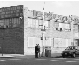
10 58-25 QUEENS BLVD This single story, 15,500sf warehouse property will soon be the home of a new 77,000sf mid-rise residential and retail property.
