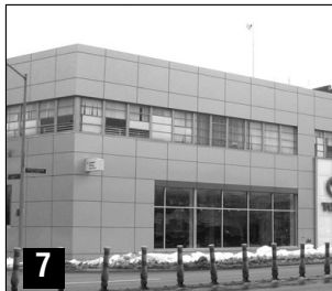
7 62-10 NORTHERN BLVD This 2-story 72,460sf industrial building had once housed a watch-band factory and publishing house. It has now been sold to Toyota as their Queens flagship location.
